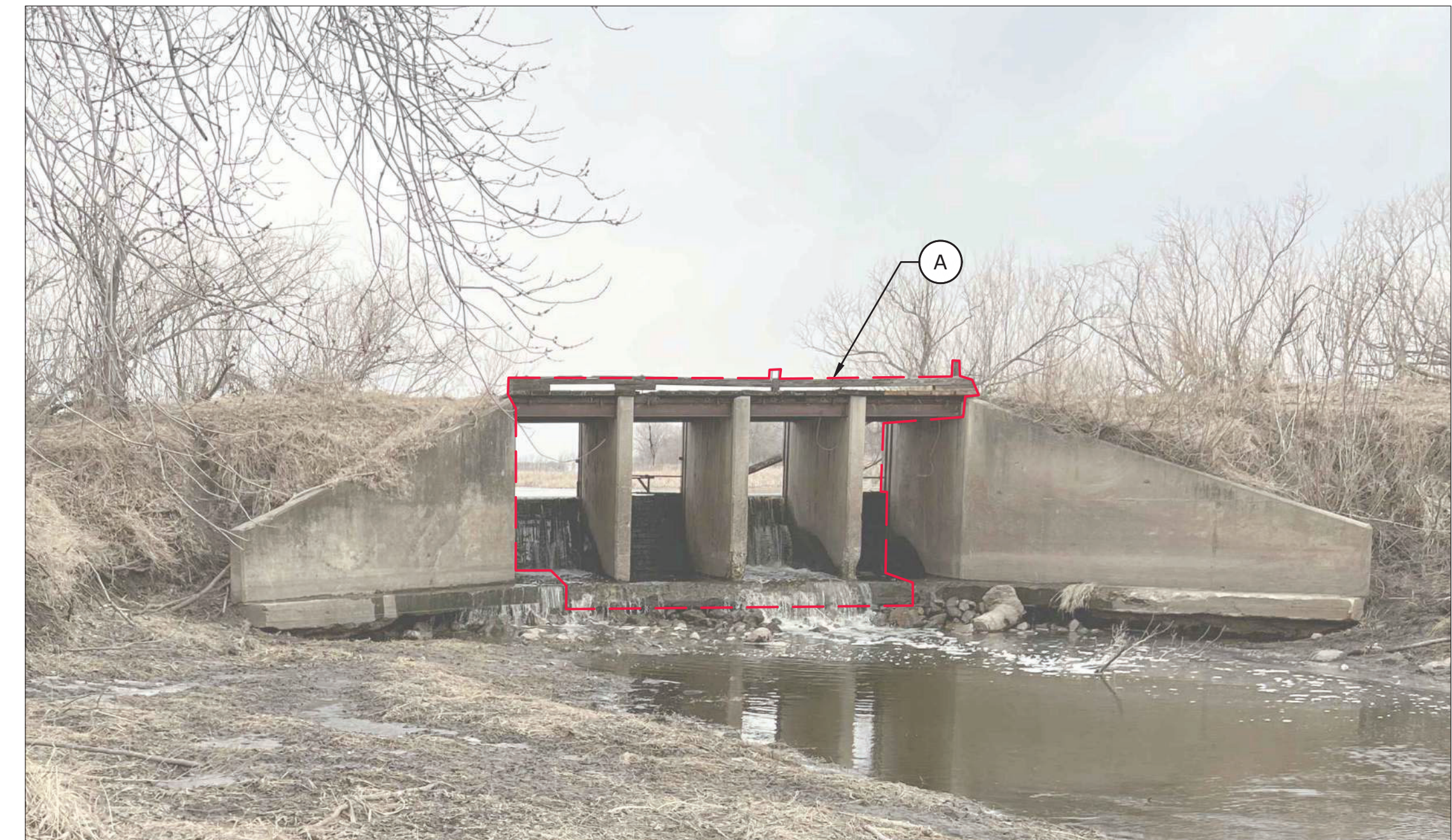
LOOKING WEST AT EXISTING LOWER STRUCTURE
