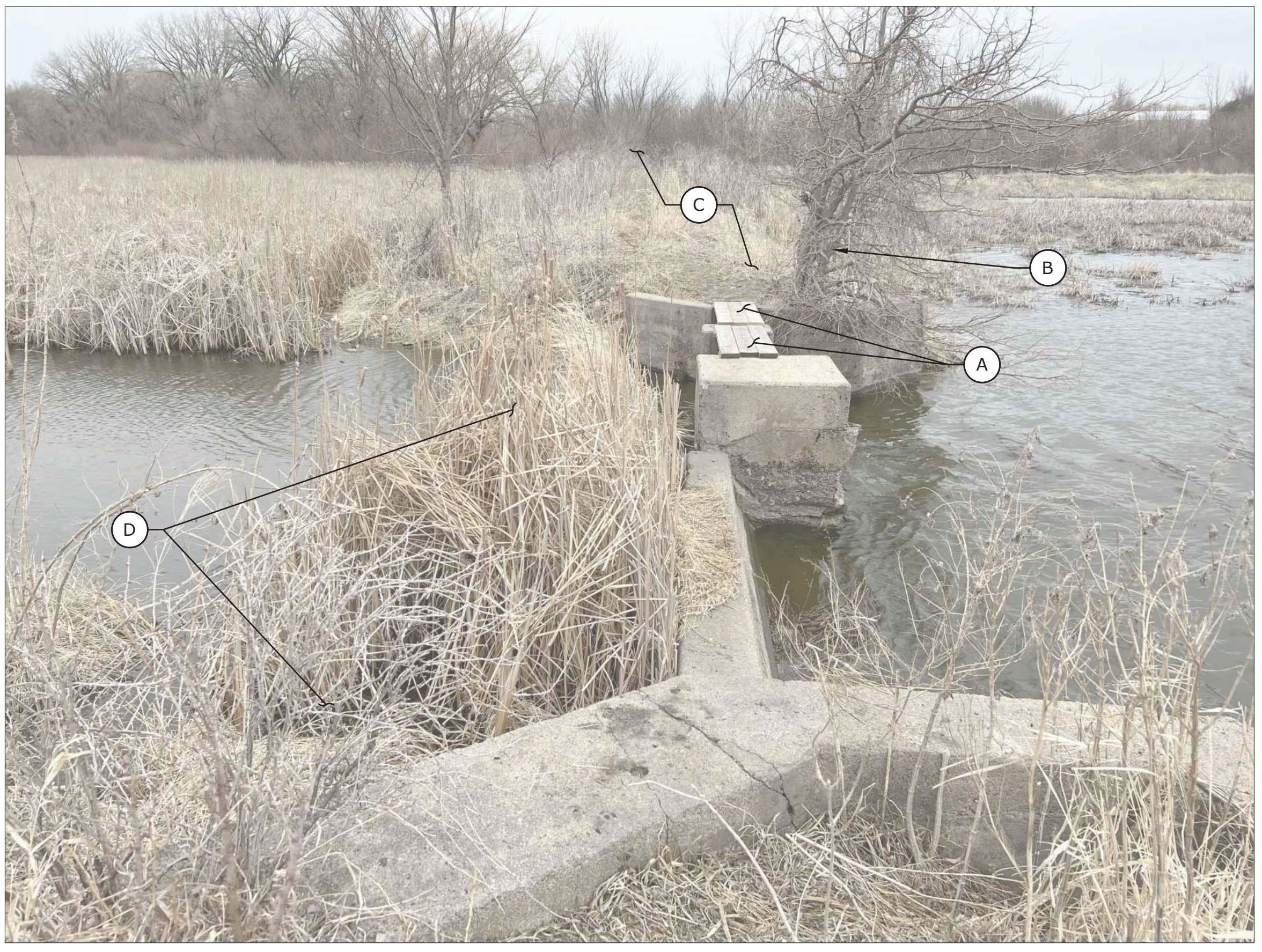
LOOKING NORTH AT EXISTING UPPER STRUCTURE
